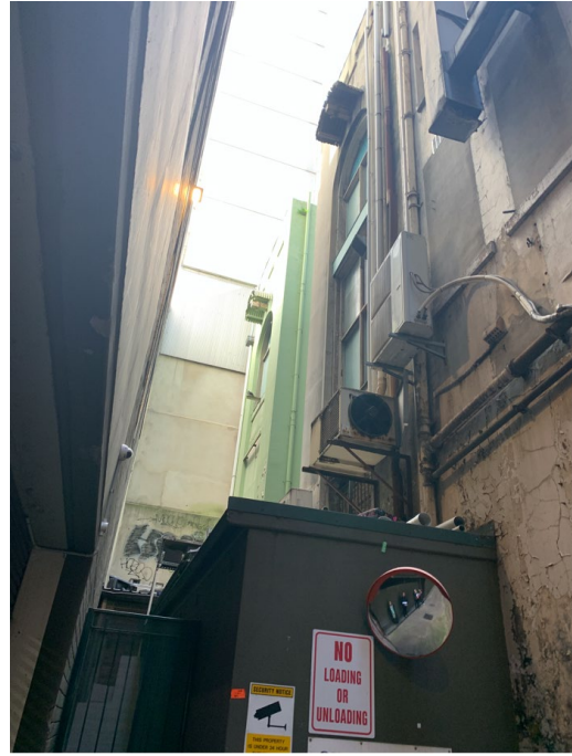
20 General view of rear of 15-17 Hunter Street
