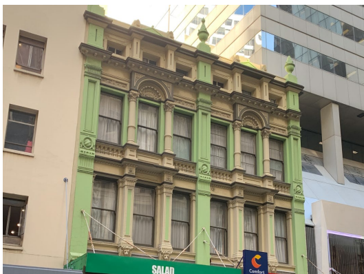
17 Detail view of upper stories Source: City of Sydney Council, August 2020
