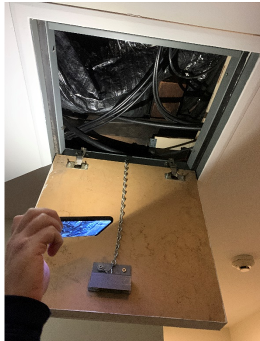
28 View into ceiling hatch appearing to show early timber roof/ceiling structure
